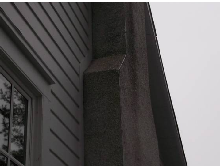
Living room chimney shoulders are stucco.
