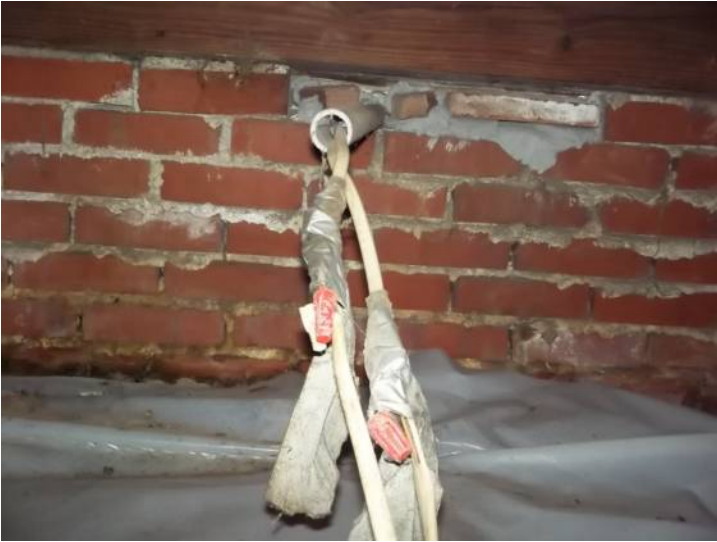
Exposed slice present in crawl space at right wall.
